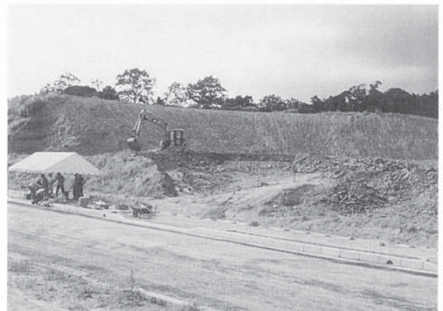
Fig. 5 The excavation site in September, 2000.
